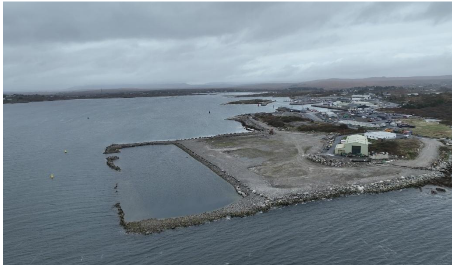
Plate 5-2: Status of the development on 29 th October 2024.
